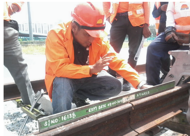
Welding preparation at Subang depot
